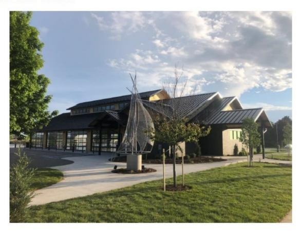
Tanglefoot Park utilized a combination Rectangular Open Gable steel pavilion with 2x6 T&G roof deck, Standing Seam metal roofing, 4x8 double T&G Northern White Cedar timber wall infill. The farmers' market event center also incorporated insulated glass garage doors, burnished cement block walls, and aluminum storefront doors and windows.
