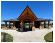
The Morgan Creek Park project in Cedar Rapids, IA is a massive 50' x 68' shaded structure held up by (16) 6" x 6" quad beam columns. The roof features a 4:12 roof pitch. The front of the shelter has an impressive 8:12 pitched dormer to welcome park visitors. The front dormer gable also features a post beam truss design. This stunning structure can shelter up to 125 people for a variety of community events.
