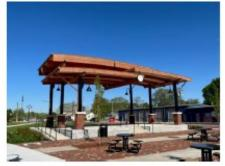
Greenfield, IN is home to this impressive, custom Wood Barrel Vault shelter. The multi-tiered structure is enhanced with its factory applied contrasting stain on the wood rafters and T&G roof decking, extra tall column height, Jet Black powder coated columns, curved wood rafter design and a Copper Penny metal roof. The striking shelter is beautiful from every angle!
